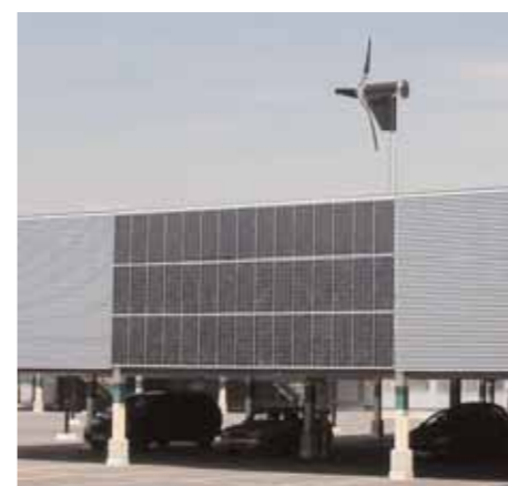
Microgrid at Croydon Central Acsolarcentury.com www.solarcentury.co.uk
